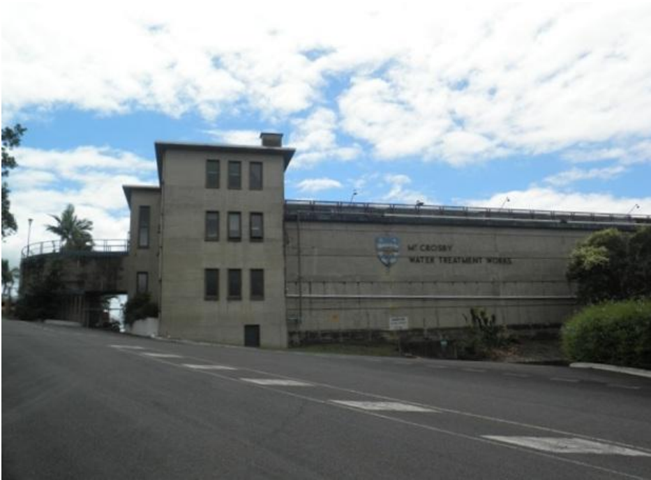
Mount Crosby Waterworks Buildings
