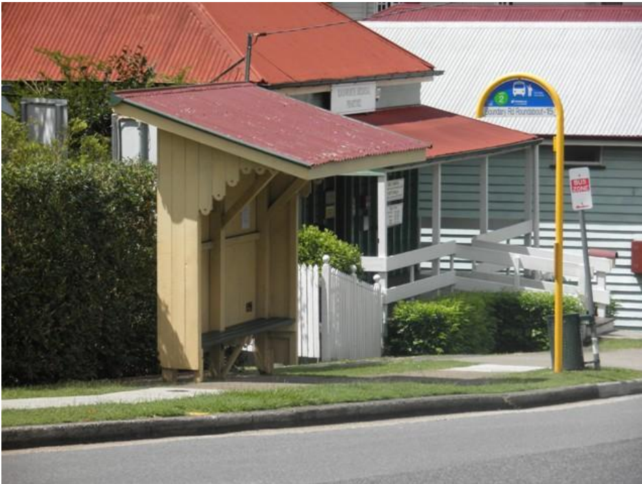
Tram Shelter No. 4 (former)
