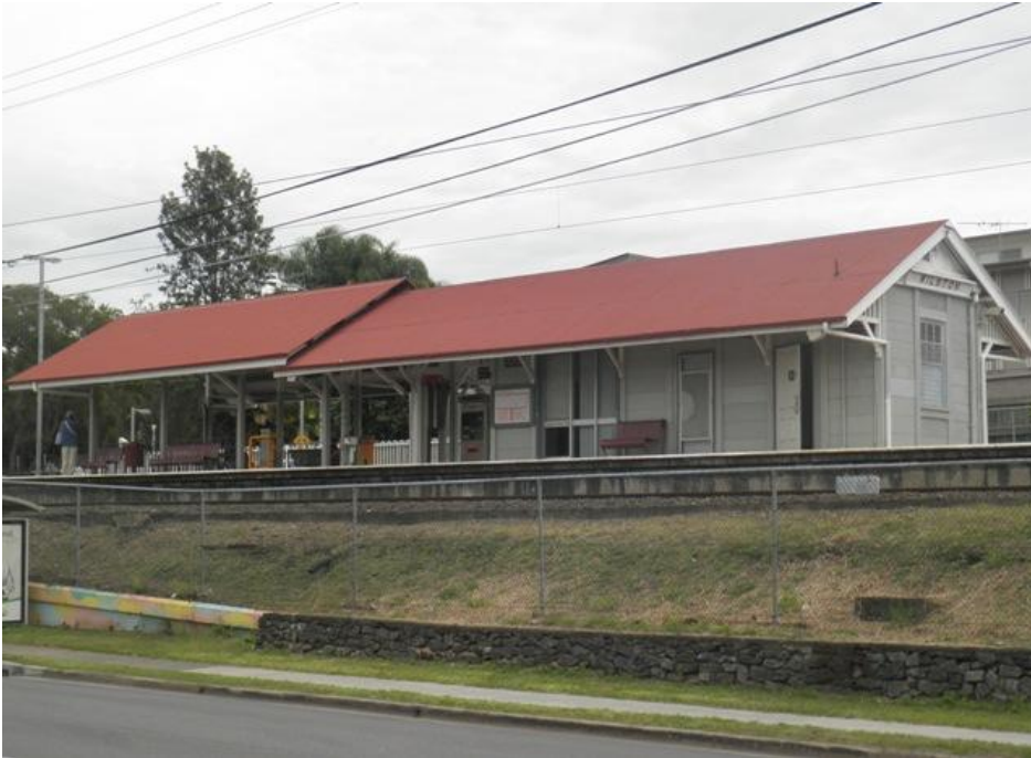
Wilston Railway Station
