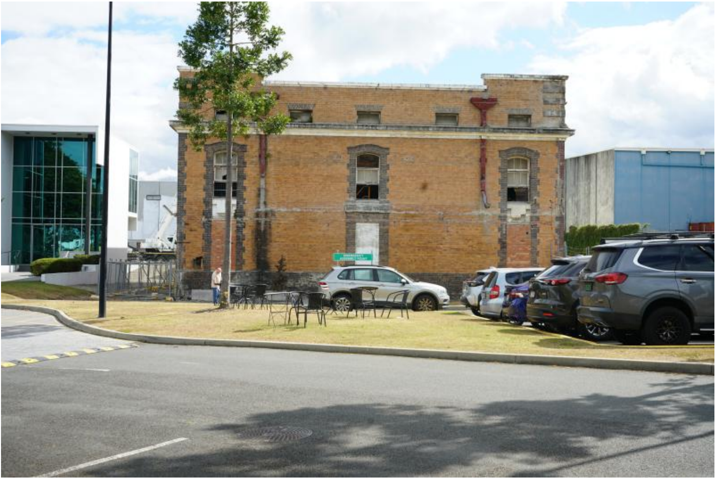
Frontal view of the Queensland Cement and Lime Company powerhouse (former).
