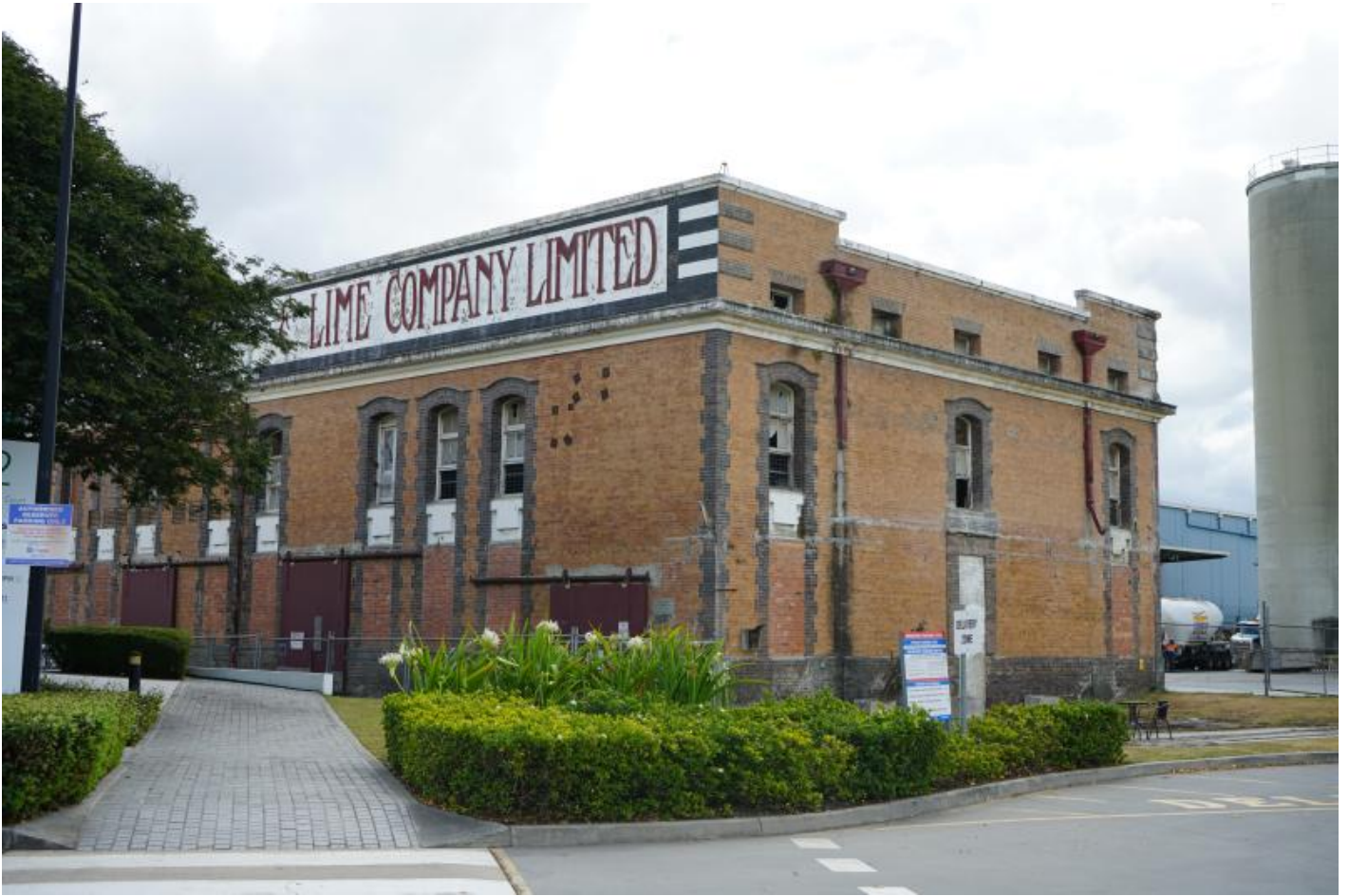
Three quarter view of the Queensland Cement and Lime Company powerhouse (former).
