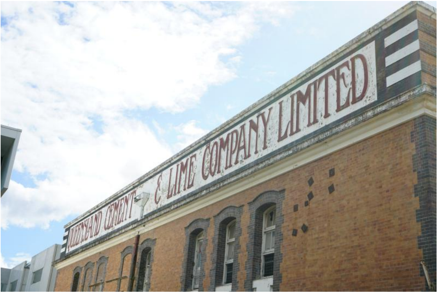
Original painted 'Queensland Cement & Lime Company' signage to the parapet.
