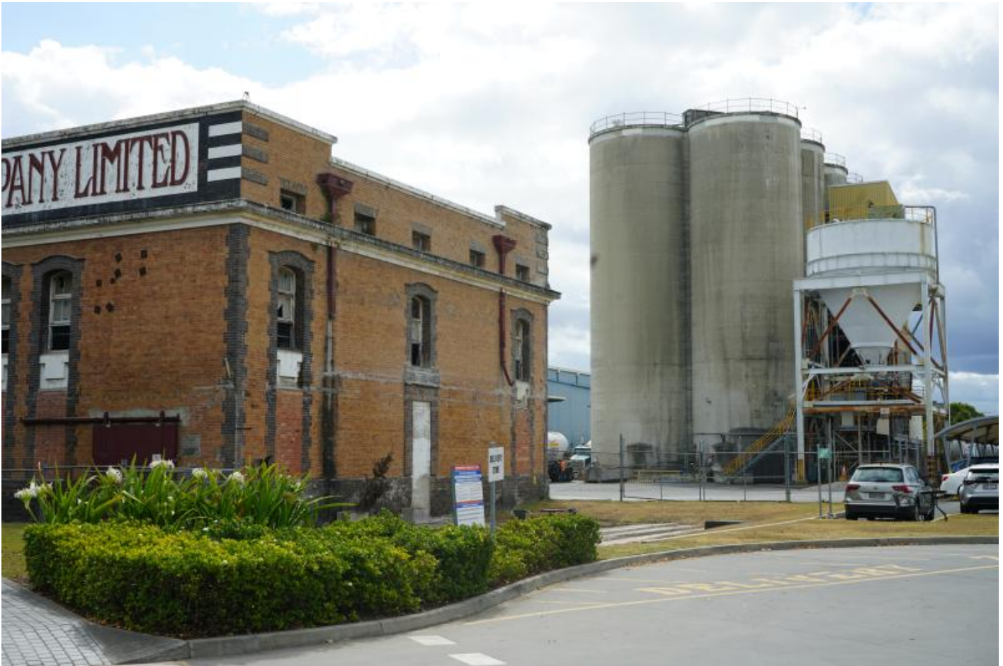
Front three quarter view of the former powerhouse with the modern cement factory in the background.
