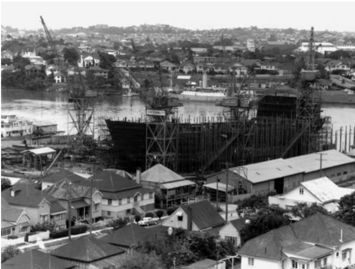
Evans Deakin Shipyards at Kangaroo Point, Brisbane, 1963 (JOL, SLQ, image number 9907). Mullen's Cairns Street cottages are in the foreground.
