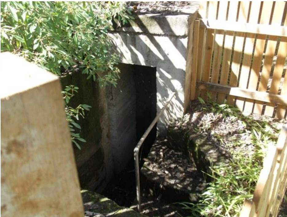
Air Raid Shelter
