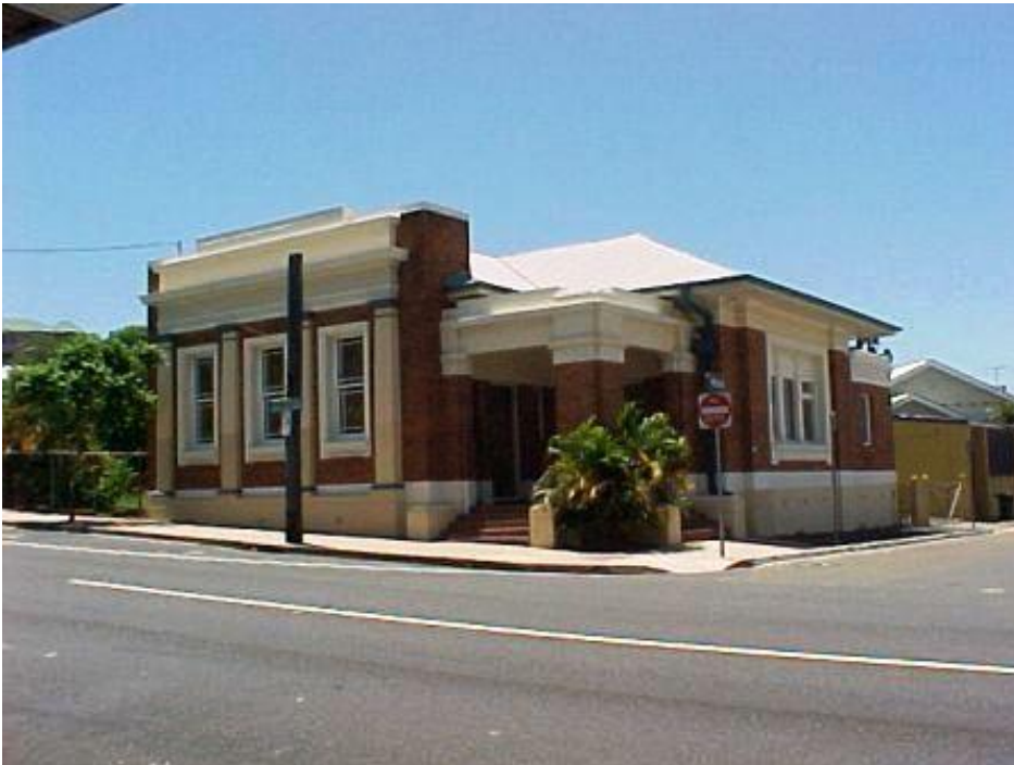
Albion Post Office (former)
