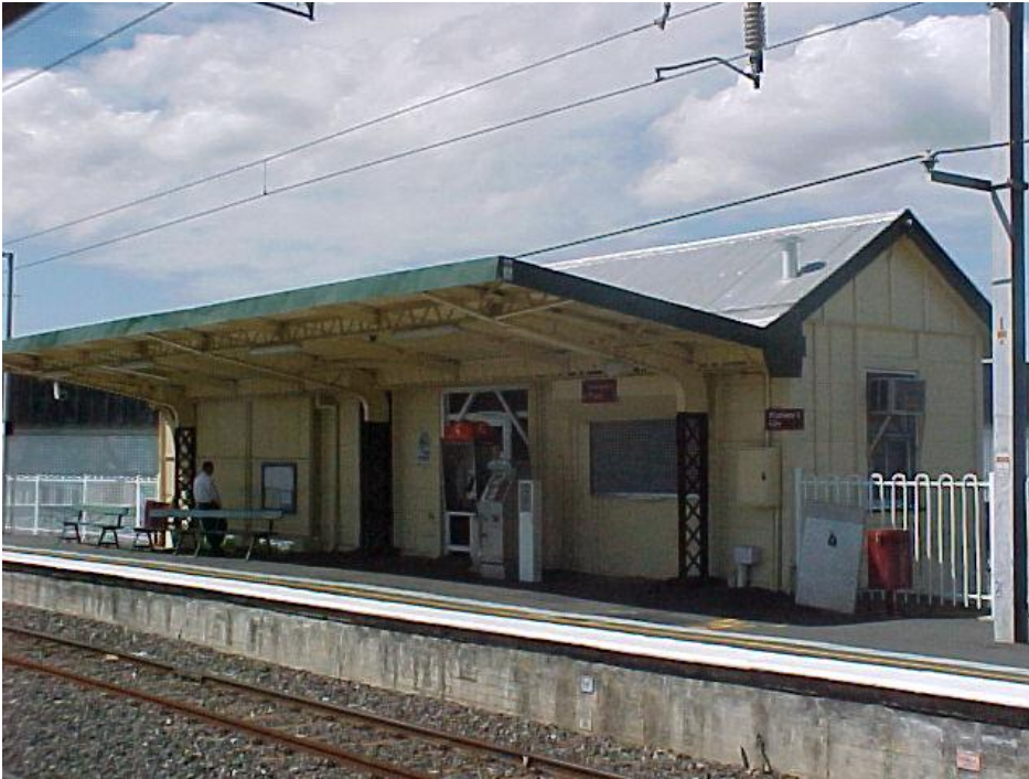
Alderley Railway Station
