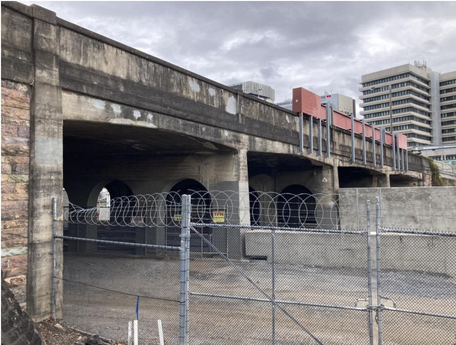
Bowen Bridge & approach walls
