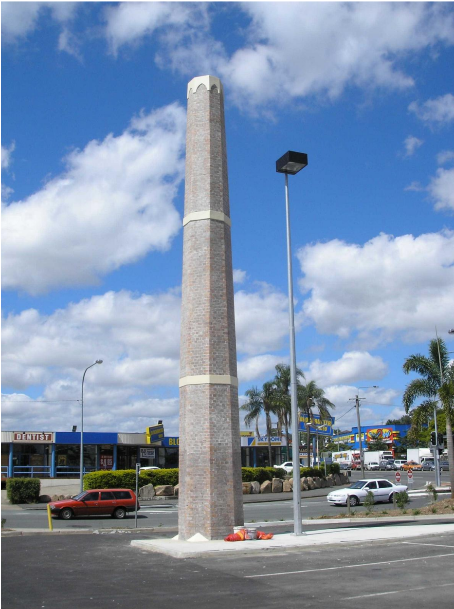
Buranda Ventilation Shaft
