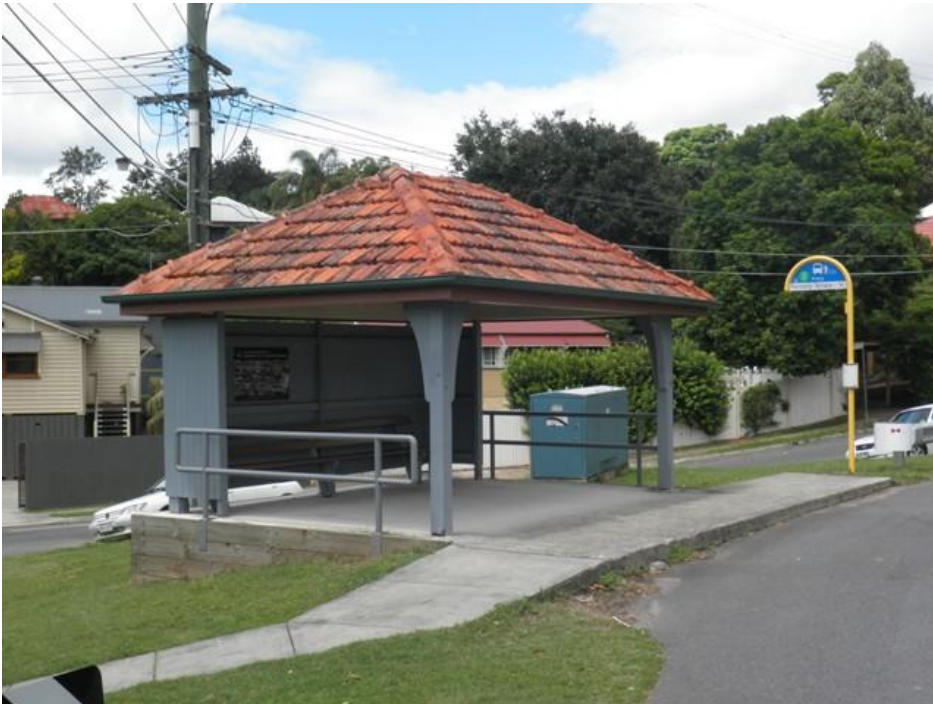
Bus Shelter No. 2
