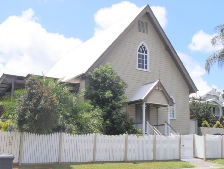
Congregational Church & Hall (former)
