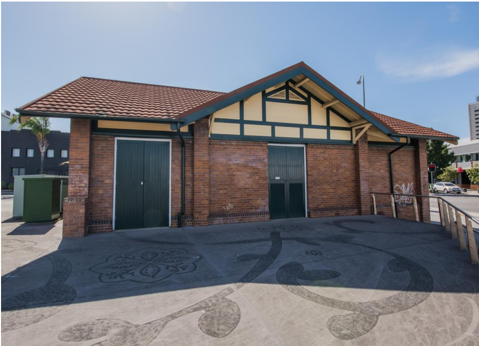
Electrical Substation No. 5
