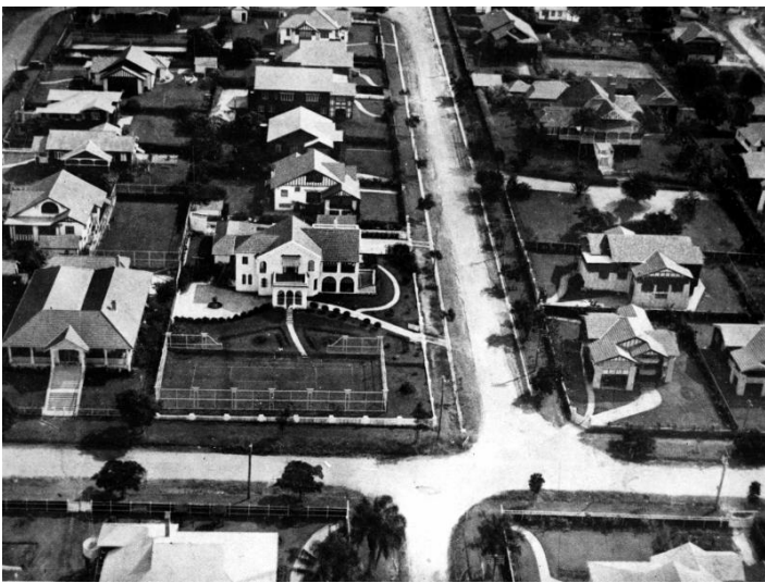
The Queenslander (Brisbane, Qld. : 1866-1939), 'Aerial view of houses in Clayfield, Brisbane, 1930', John Oxley Library, State Library of Queensland
