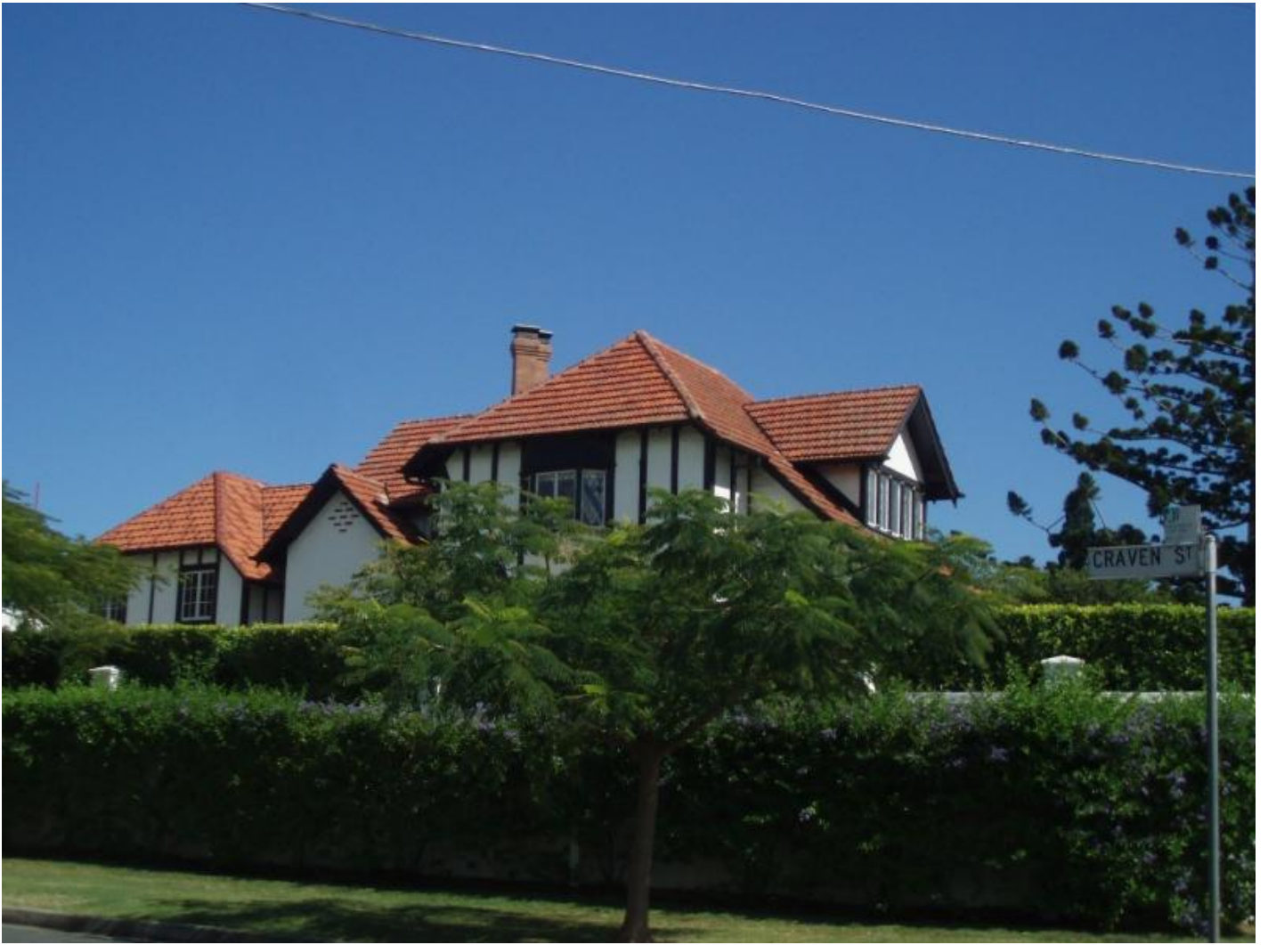
Delcotta, 19 Craven St, (was 51 Enderley Rd) (1645 m 2 )
