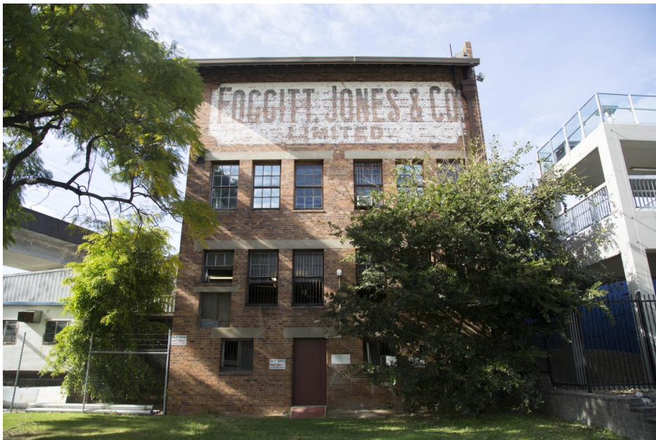
Foggitt & Jones Factory (former)
