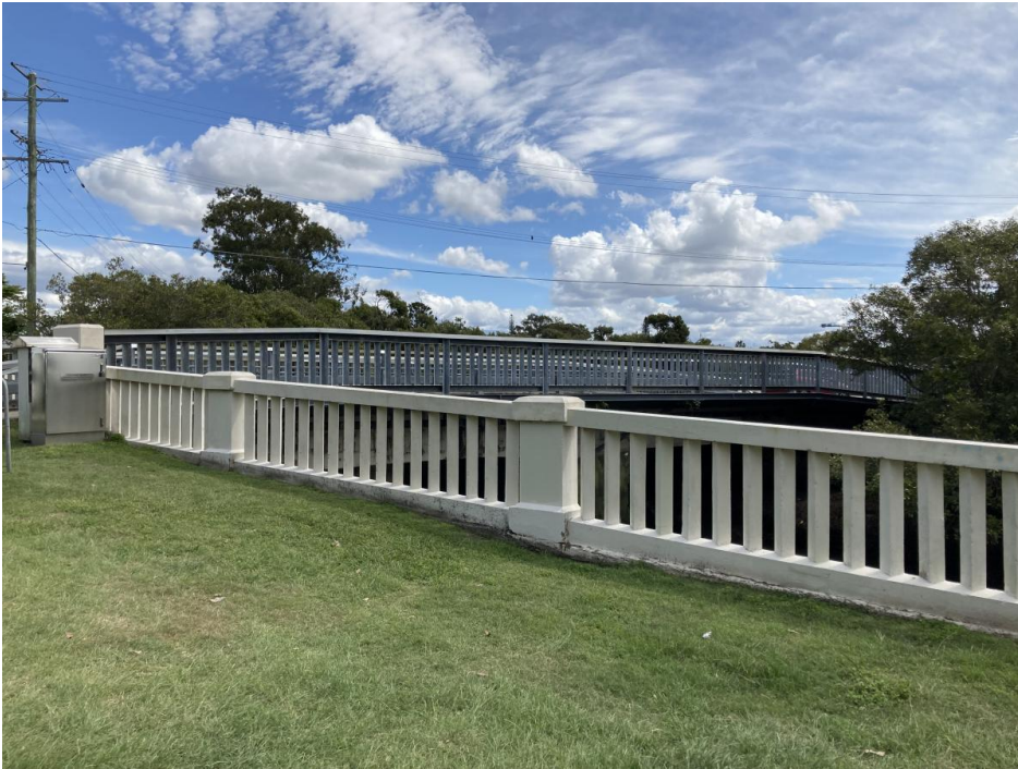
Fox Street Bridge
