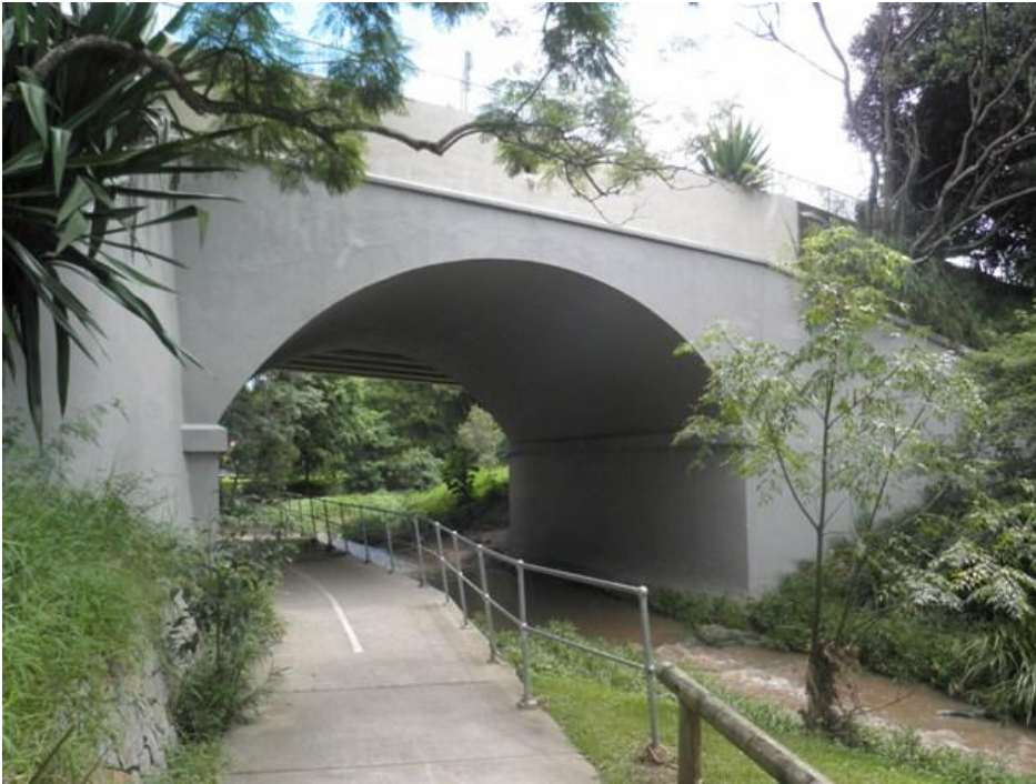
Ithaca Bridge (near Mossvale Street)
