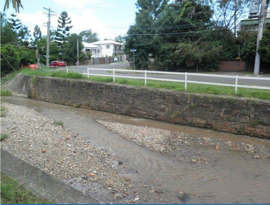
Ithaca Creek Stone Embankment
