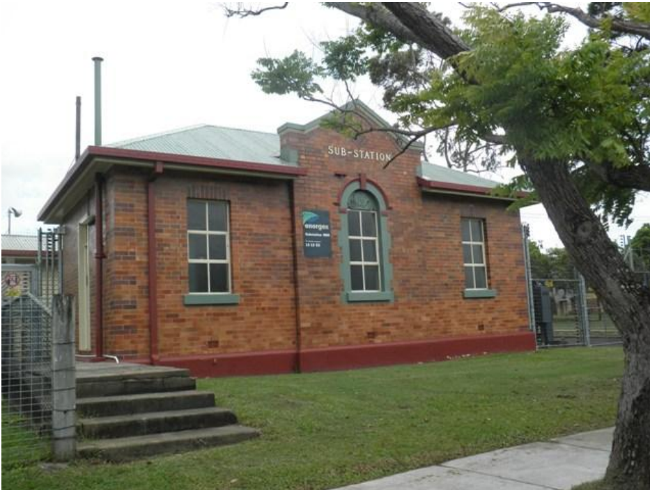
Nundah Substation No. 237
