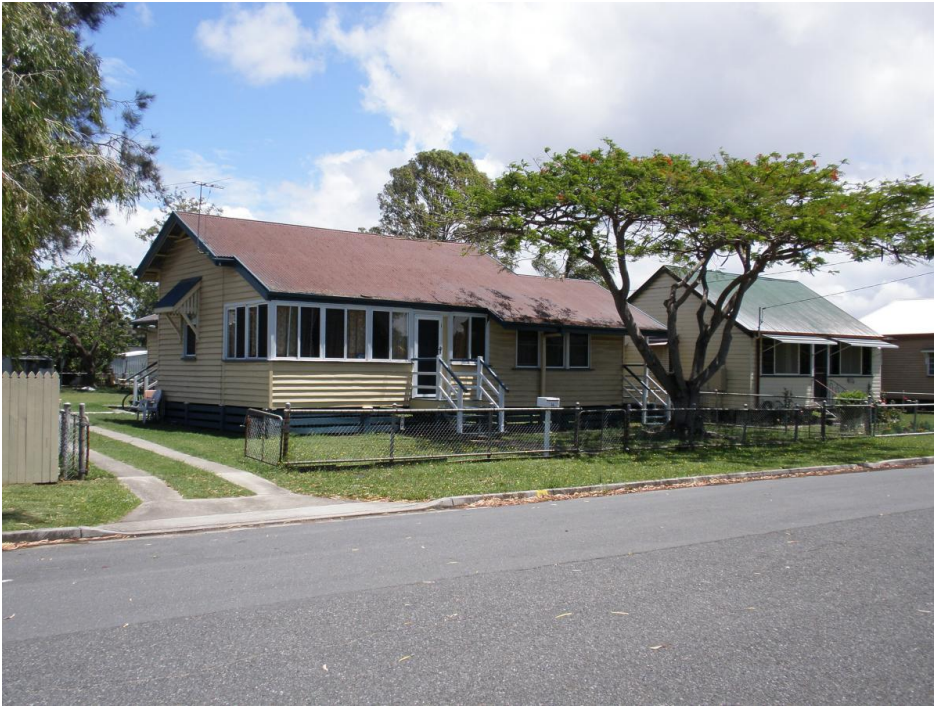
Pinkenba Police Station (former)
