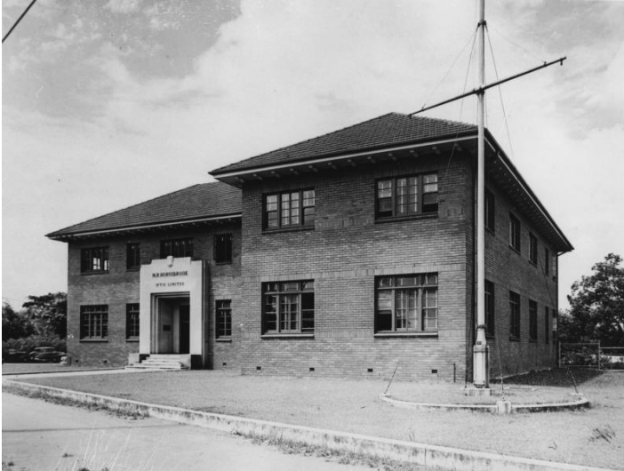
The Green Studio, H.B. Green & Co. (photographer), 'Headquarters of M.R. Hornibrook (Pty) Limited in Newstead, Brisbane, ca. 1945', John Oxley Library, State Library of Queensland.
