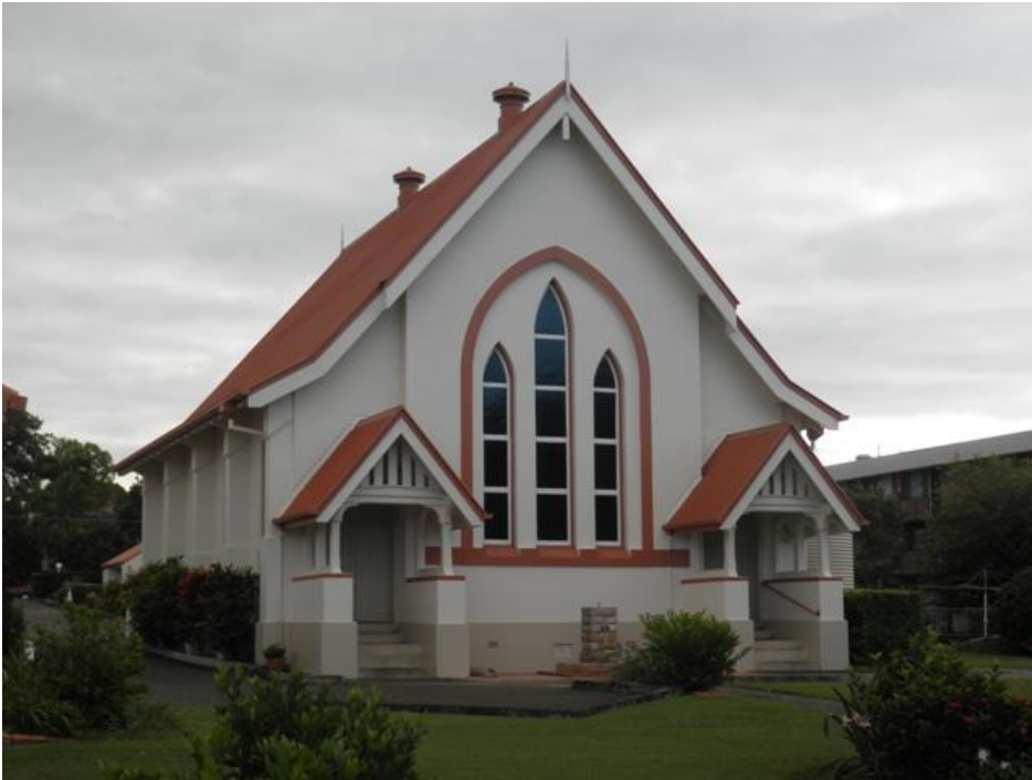
Sherwood Presbyterian Church (former)
