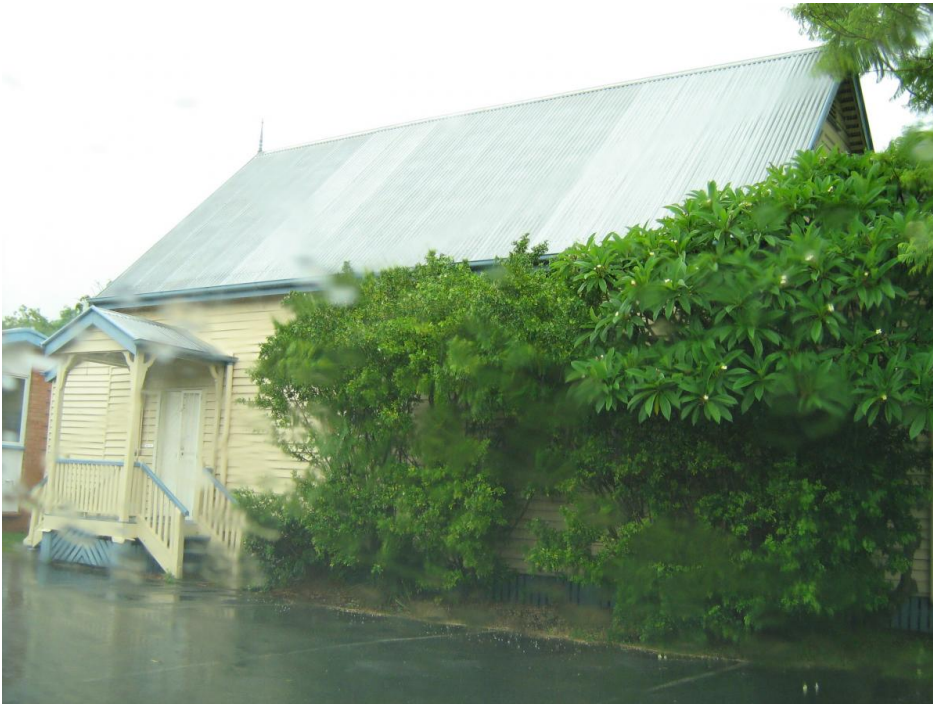
St Peters Church (former)
