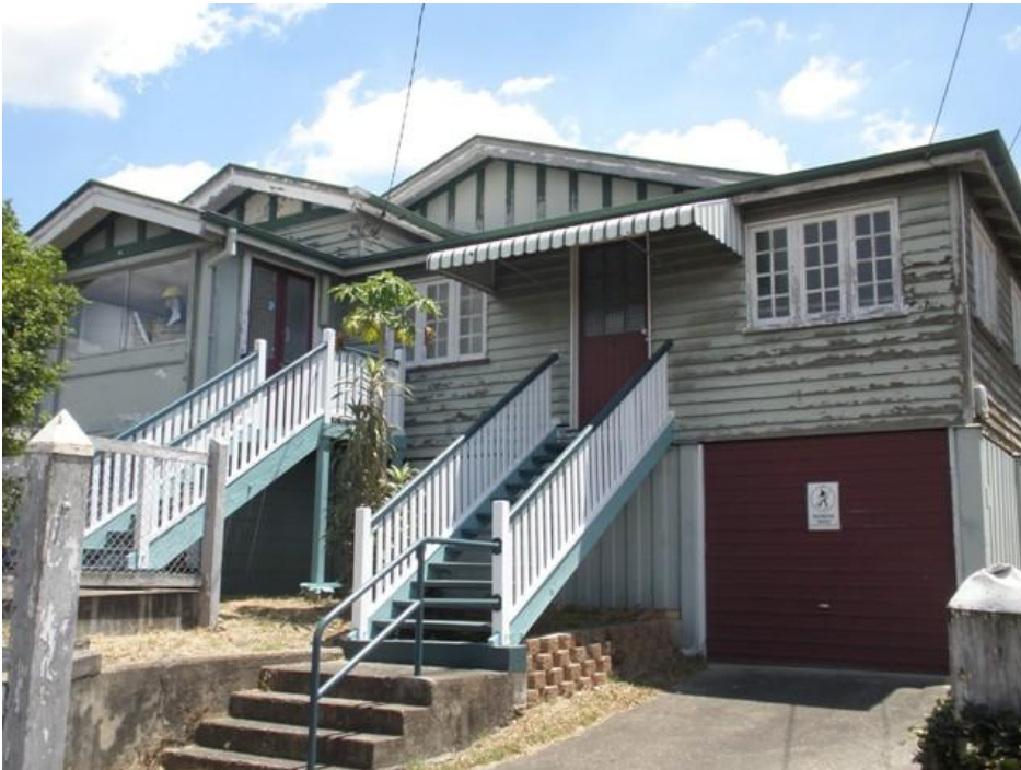
Torwood Police Station
