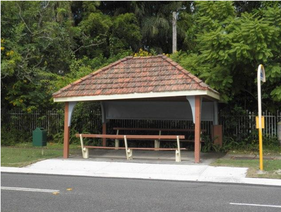
Tram Shelter (former)
