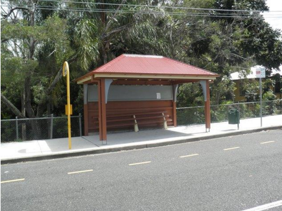
Tram Shelter No. 1 (former)
