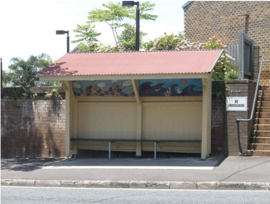
Tram Shelter No. 3 (former)
