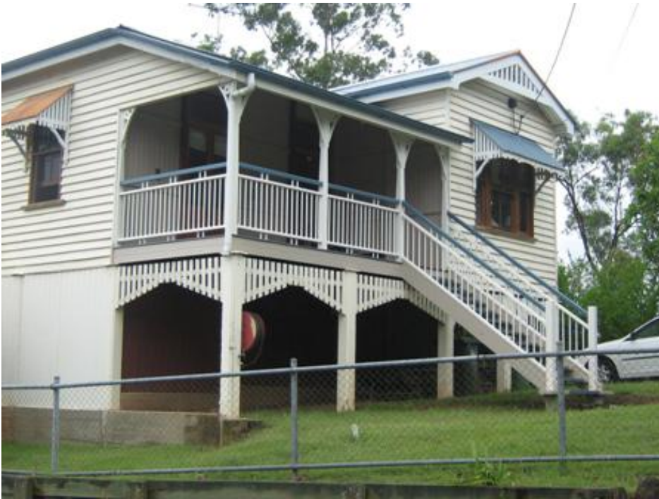
Waterworks Cottage No. 117
