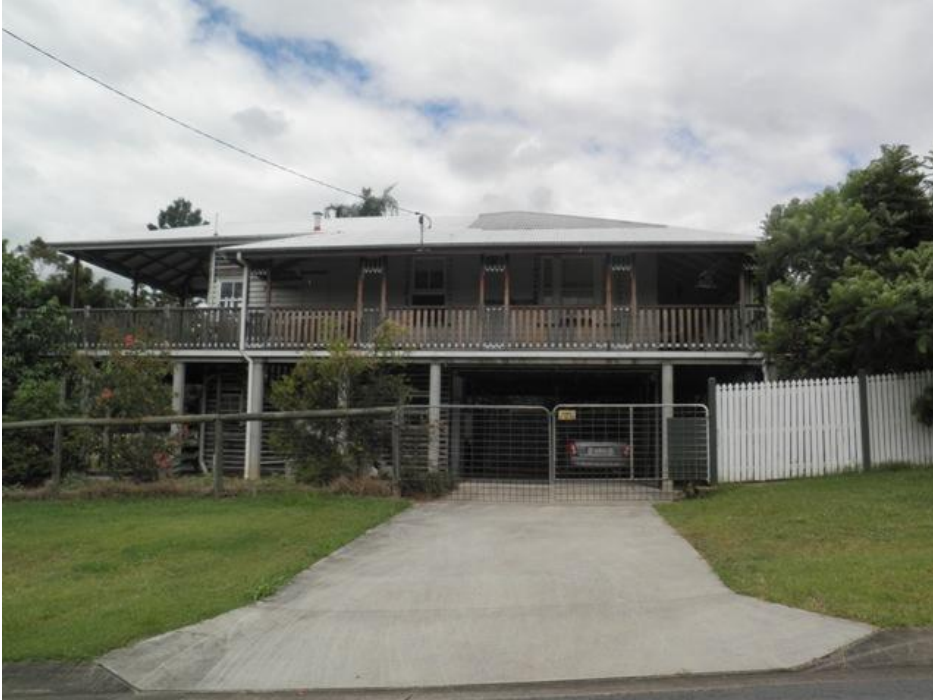
Waterworks Cottage No. 121
