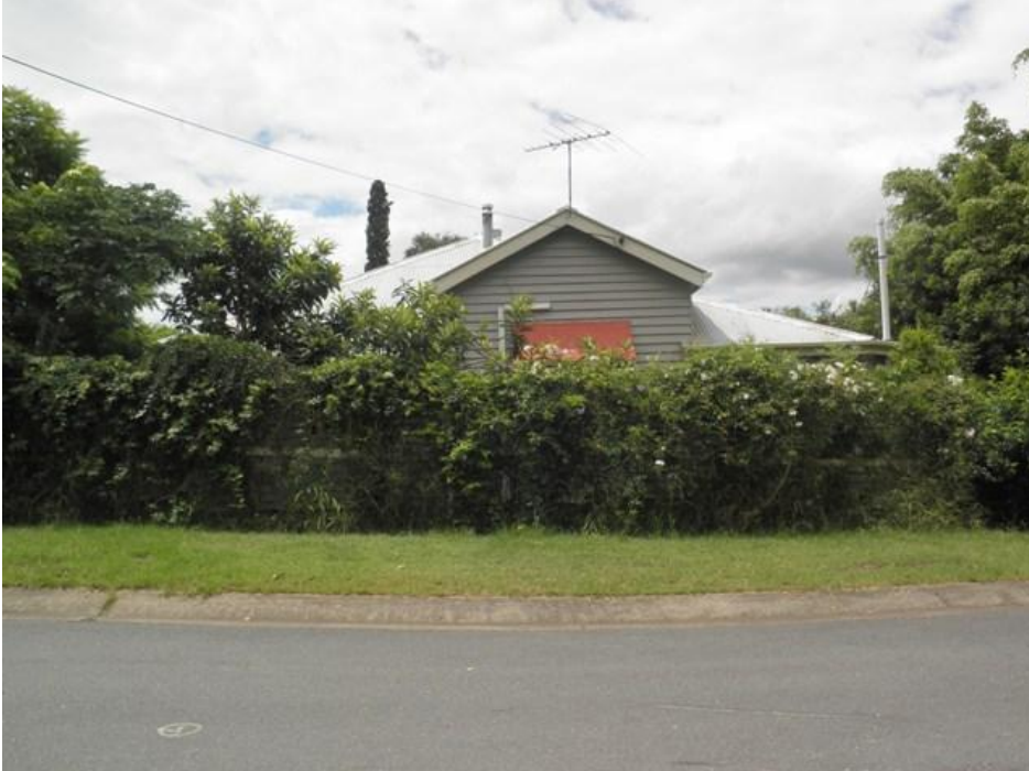
Waterworks Cottage No. 122
