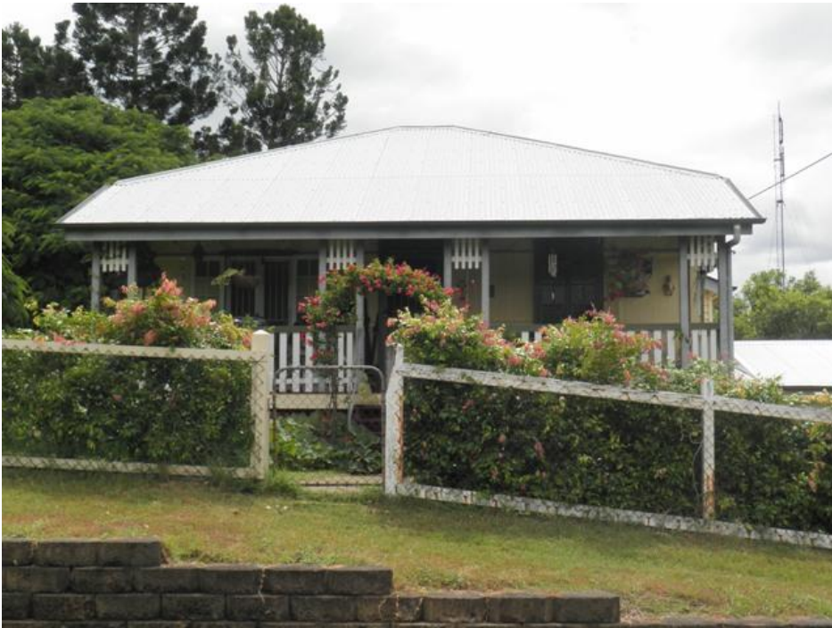
Waterworks Cottage No. 130
